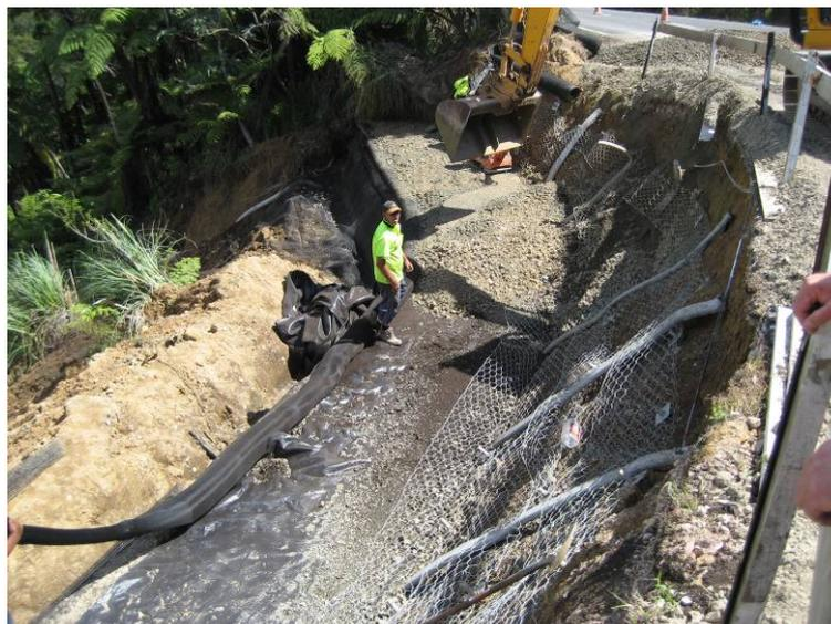
**Figure 3:** Construction stage showing connection between LSNs and GCS backfill
