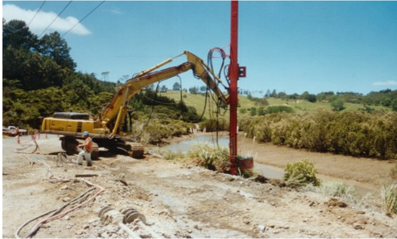
Figure 5. Installation of columns
