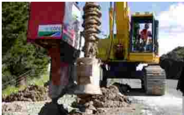
Figure 2. Close-up of the counter-rotating auger head assembly
