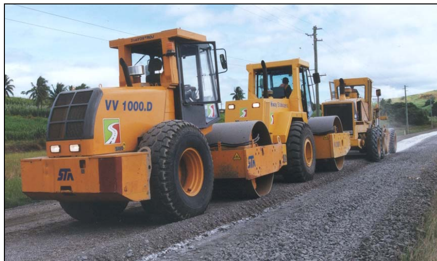
Photo 4: Twin smooth drum rollers following basecourse stabilising.
