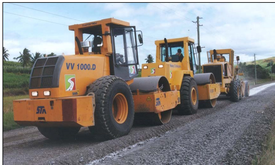
Photo 4: Twin smooth drum rollers following basecourse stabilising.
