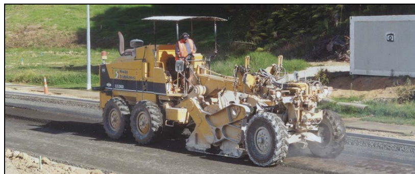
Photo 2: Basecourse stabilising – Komatsu GS 360 Hoe.
