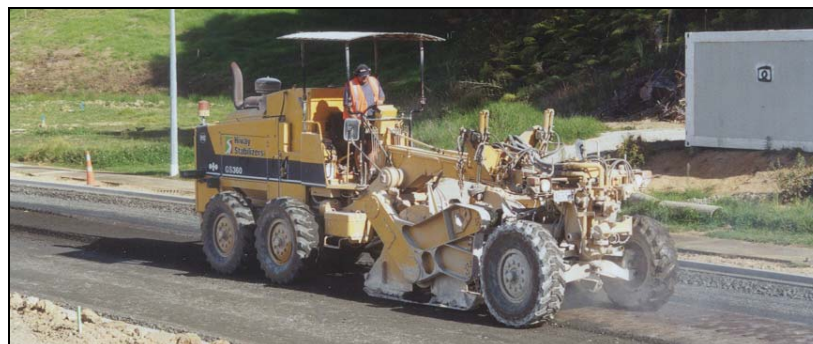
Photo 2: Basecourse stabilising – Komatsu GS 360 Hoe.
