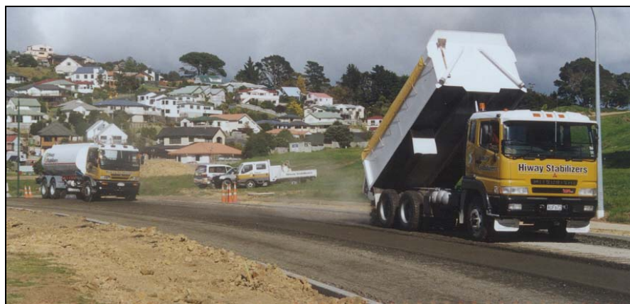
Photo3: Spreading KOBM followed by water cart for basecourse stabilising.
