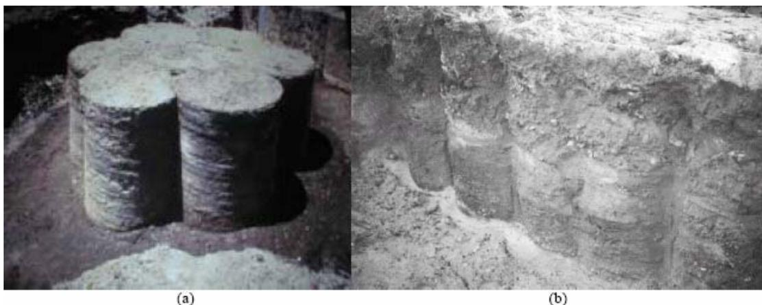
**Fig 1. Examples of columns created using deep soil mixing augers: (a) overlapping configuration (photo SMW Seiko, 1997) and (b) barrier wall configuration (photo May Gurney Technical Services, 2001) (Al-Tabbaa A, Perera A.S.R 2002a)**
