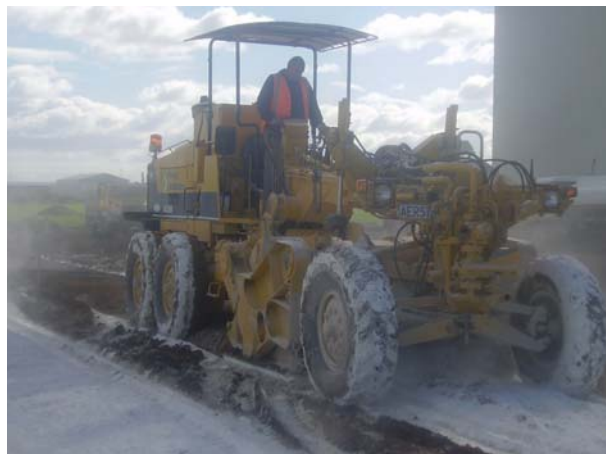
Figure 6.1: Field trial stabilisation underway.
