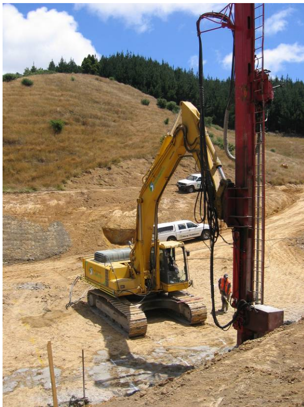
Figures 7 and 8: Construction of Colmix columns
