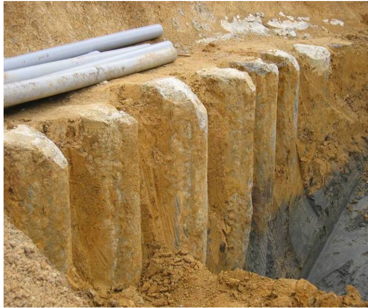
Figures 9 & 10: Photos showing exposed trial columns
