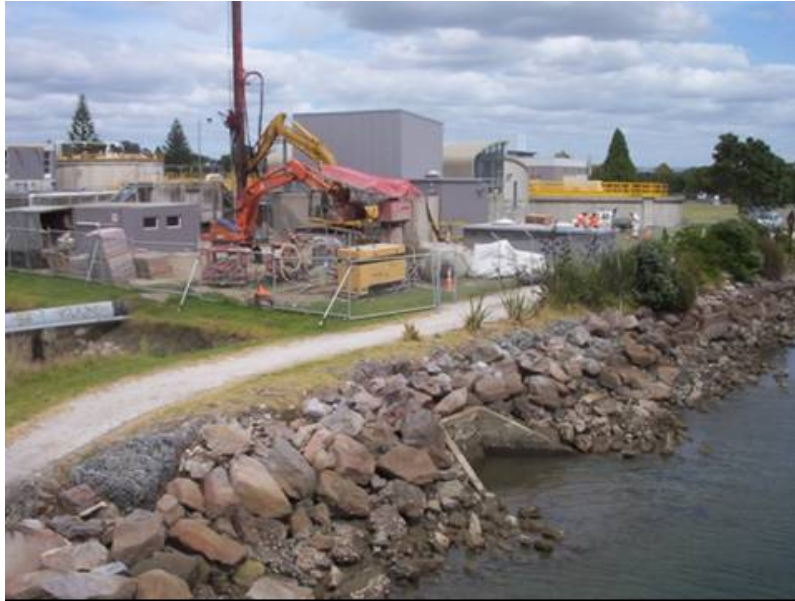
Photo 1: Ground improvement site.
