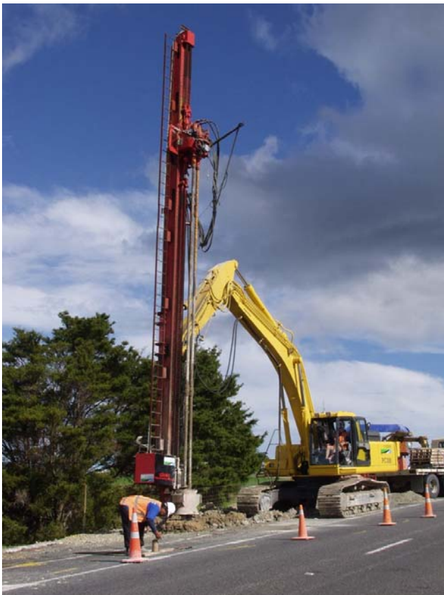
Figure 3: Colmix rig
