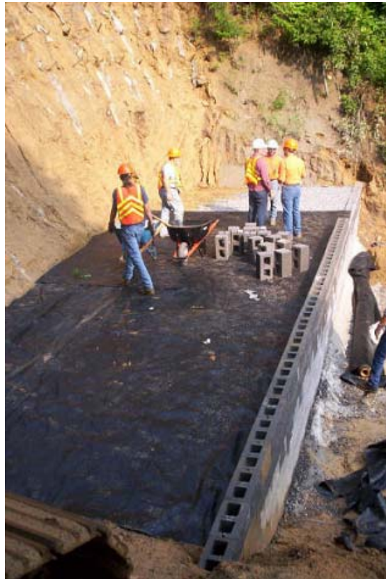
Figure 12. GRS wall being constructed on launched micropiles
