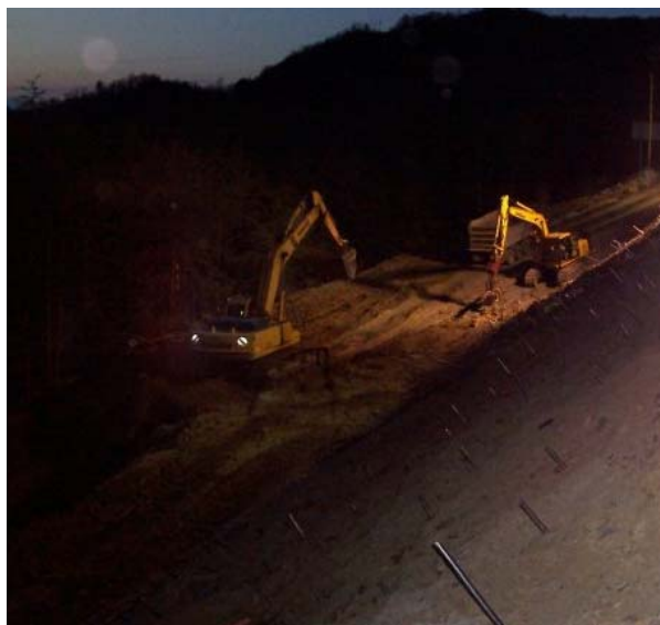
Figure 9. Excavating trying to keep ahead of launched nailing.
