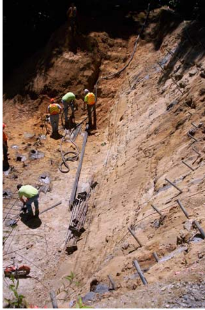
Figure 11. Launched soil nails and micropiles.
