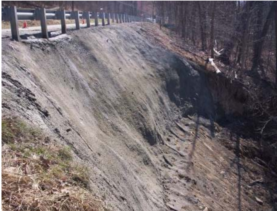
Figure 14. Shotcrete facing after launched soil nails.
