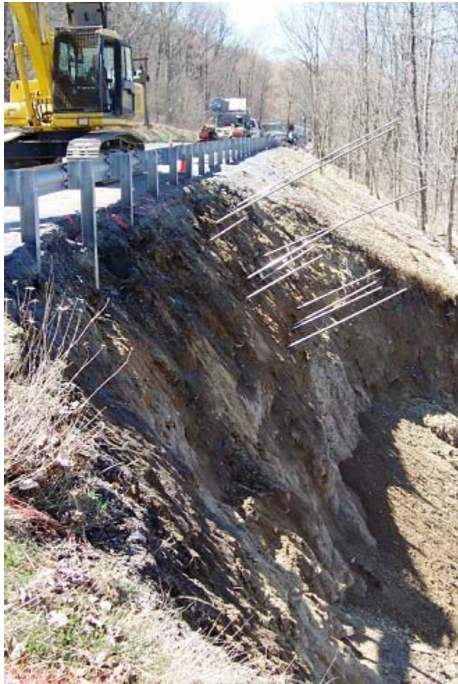
Figure 13. First soil nails launched.
