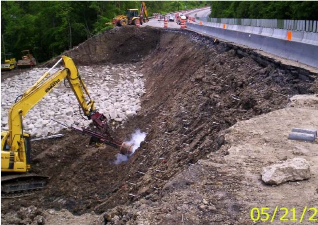
Figure 15. Launched soil nailing keeping ahead of embankment reconstruction.
