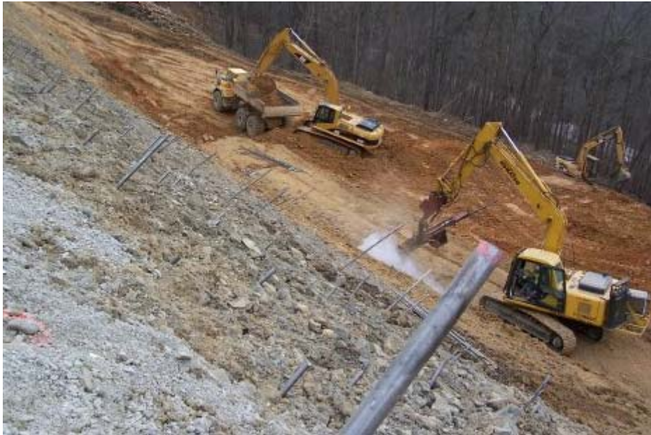
Figure 8. Excavation and nail launching working in sync.
